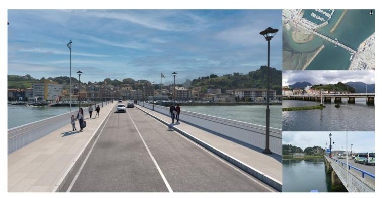
FHECOR, in JV with NOEGA Ingenieros, has prepared the draft project consisting of the complete substitution of the deck and its widening together with the support to maintain the traffic operation level during the works of construction, repair, reinforcement of the bridge substructure and the widening of the road traffic accesses. Furthermore, the project also includes the improvement of the accessibility of the nearby accesses according to current standards.
